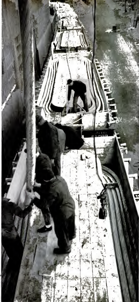
LAST LENGTH of the 39,200-foot cable is coiled into the ninth gondola car of special train. The cable
